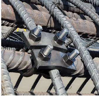
Fig. 10. Bending of the U-bolt connector plates in a tight-fit connection.
