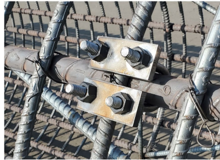
An assembled U-bolt connection on a cross-bar connection in a rebar cage
